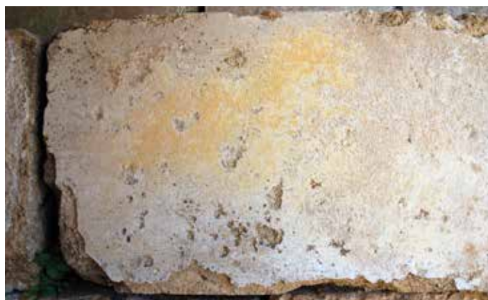
Figure 1: Lowest step of krepis on W front (third block from the north) with white plaster and yellow color on top. Photograph by James Conlon.
